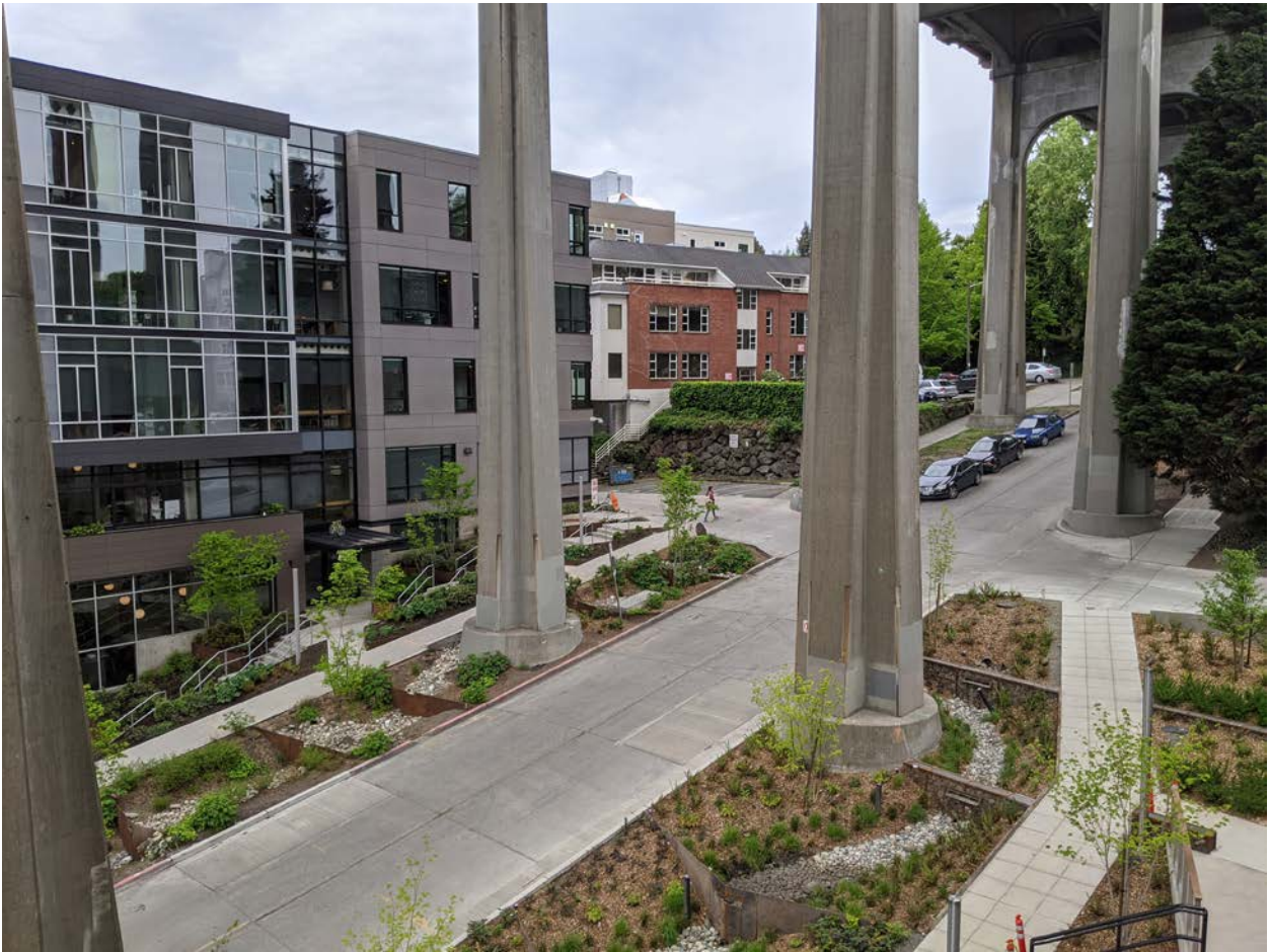
Bioswales outside Watershed filter polluted water coming off the Aurora Bridge before it reaches a nearby lake.
