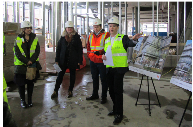
CoreNet Tour of Data I office building in Fremont, 2016
