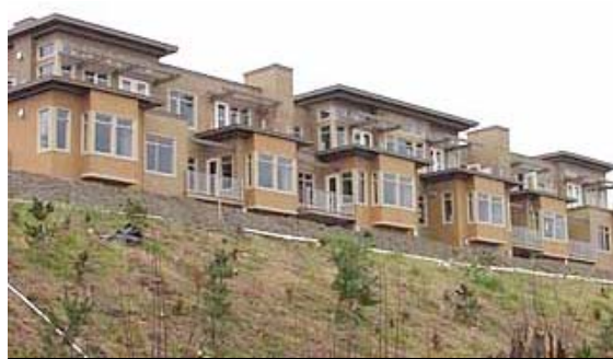
Photo by Terry Stephens Lots for the Point Edwards condos were cut into a hillside overlooking Edmonds. The tricky part was installing the project's utilities on the steep site.
